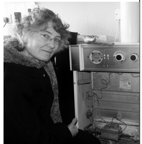
Fiona Hall MEP with an out-of-date boiler which needs replacing
